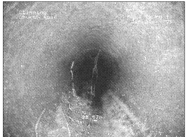
Photo: 121_6a 20.17m, Settled deposits fine 10 % cross-sectional area loss
