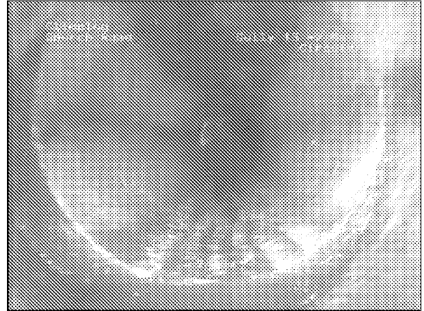
Photo: 97_3a 2.26m, Open joint medium
