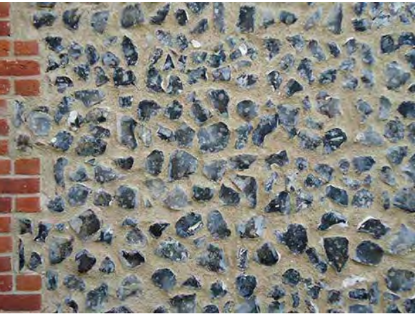
Flint blocks To match houses on Climping Street
