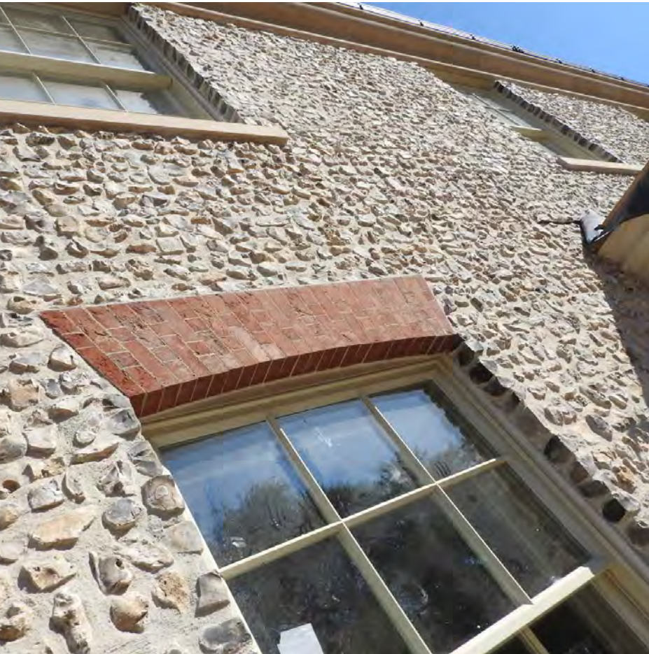
A closer look at the flint elevations on Mayfield House. Mayfield House Photography by All Brick & Stone Ltd.
