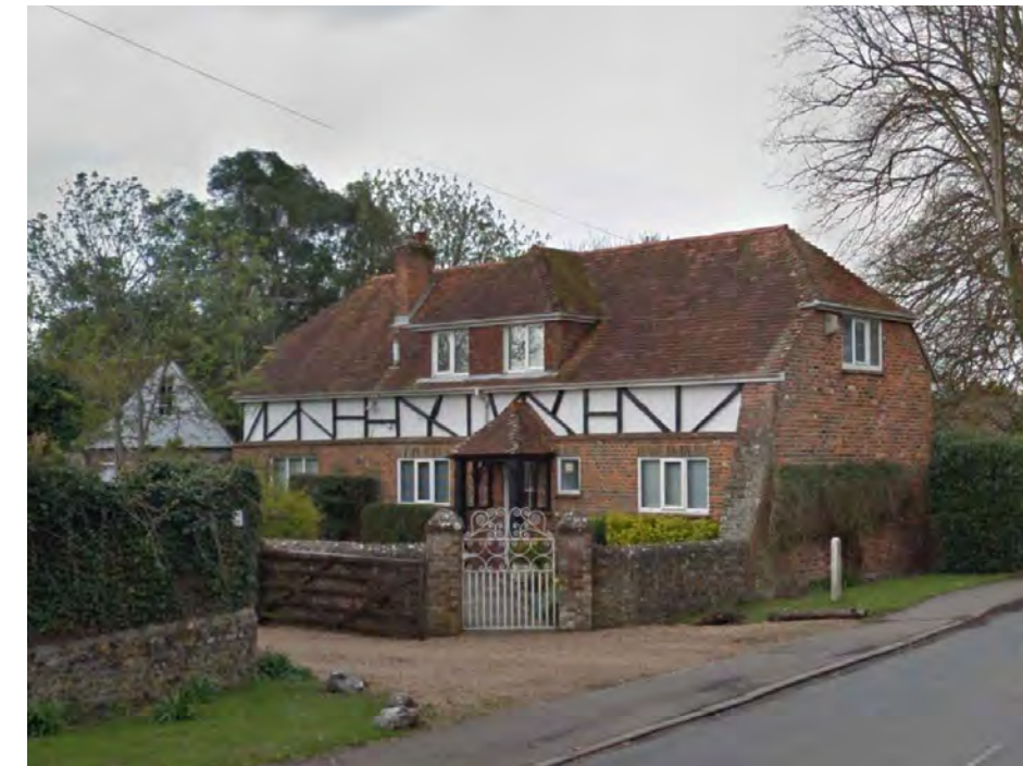
Local Precedent: The Barn, Horsemere Green Lane
