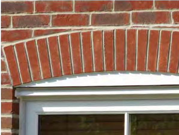
Arched headers in alternate brick
