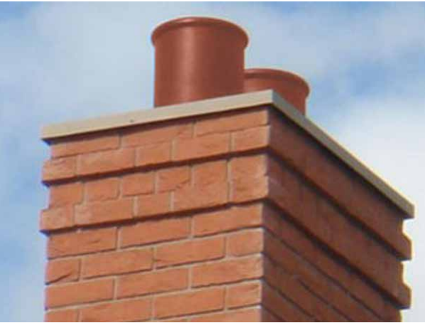
Chimneys in matching brick
