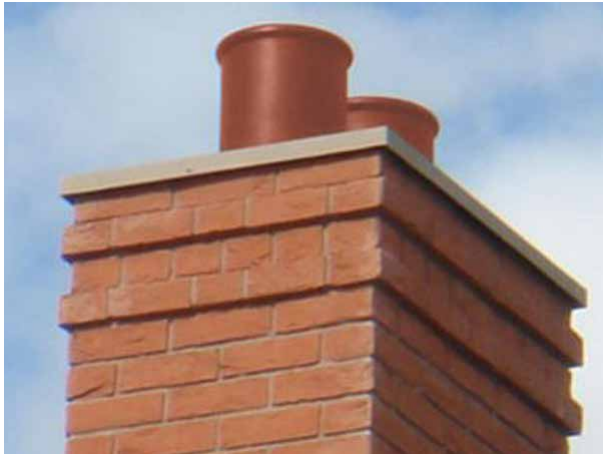
Chimneys in orange/red brick
