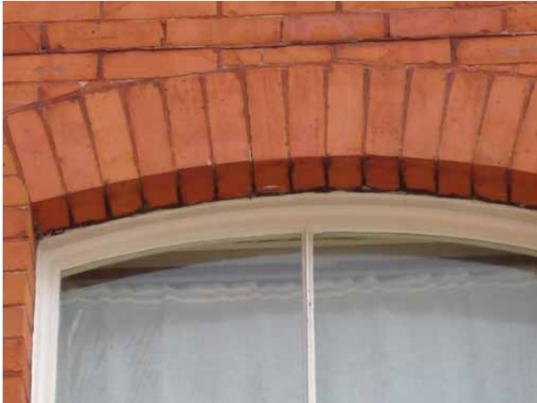
Arched headers in matching brick
