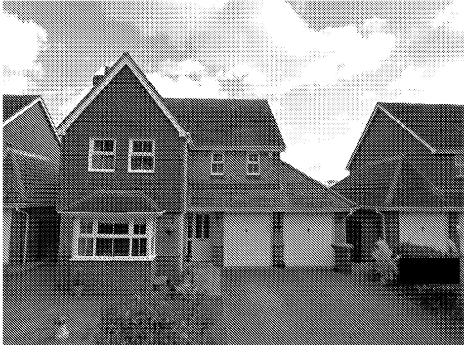
House with red tile hanging to feature gable
