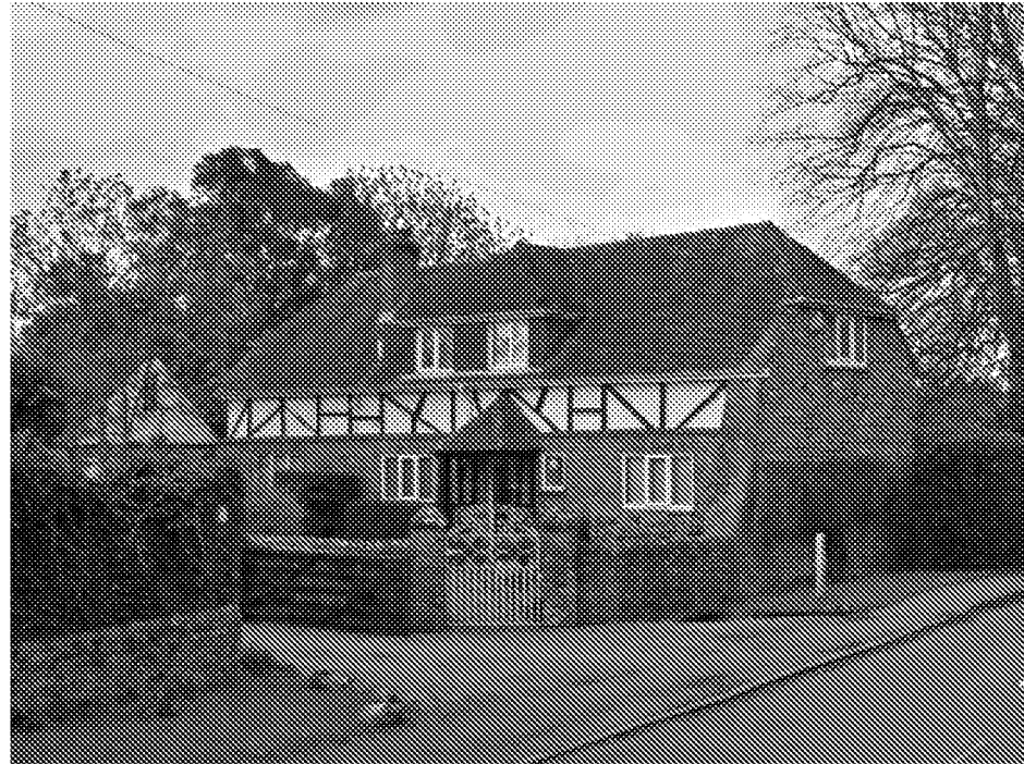
Local Barn Conversion - Horsemere Green Lane
