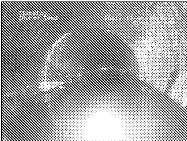
Photo: 98_4a 2.9m, Water level 50 % height/diameter
