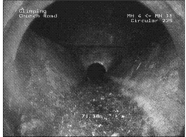
Photo: 129_14a 71.3m, Finish node type, manhole, reference number: MH 11
