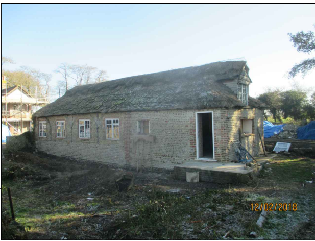
PHOTO IMAGE SHOWING EVIDENCE OF EXTREMELY POOR CONDITION OF THATCHED ROOF. PROPOSED TO BE REPLACED WITH NEW THATCHED ROOF
