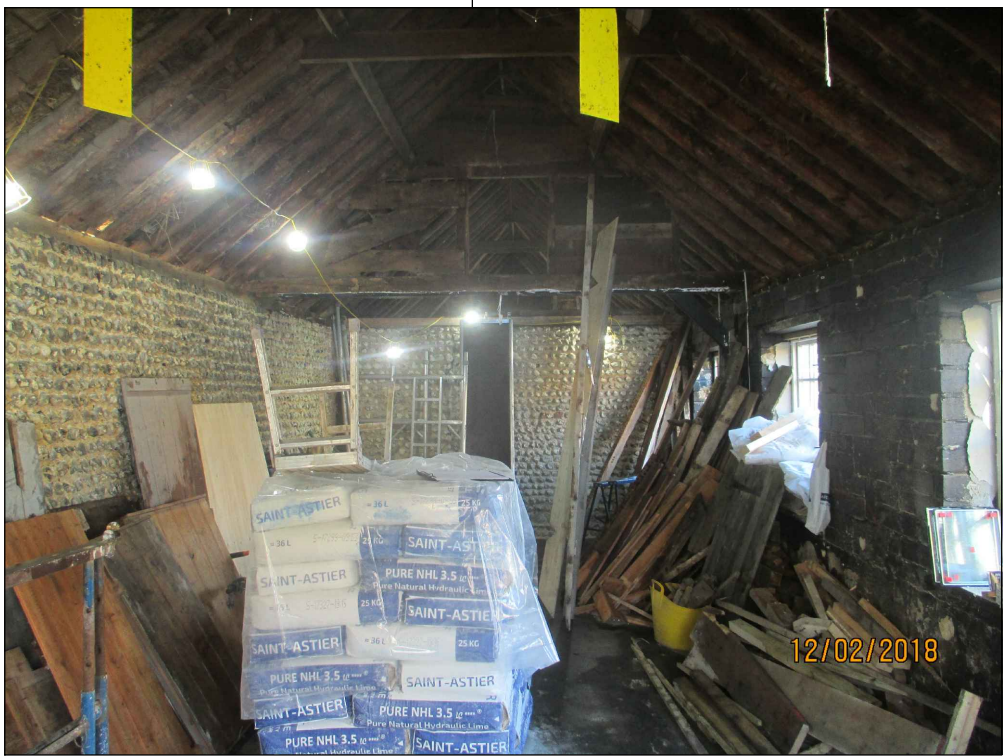
PHOTO IMAGE SHOWING EVIDENCE OF PREVIOUS MEZZANINE FLOOR LEVEL
