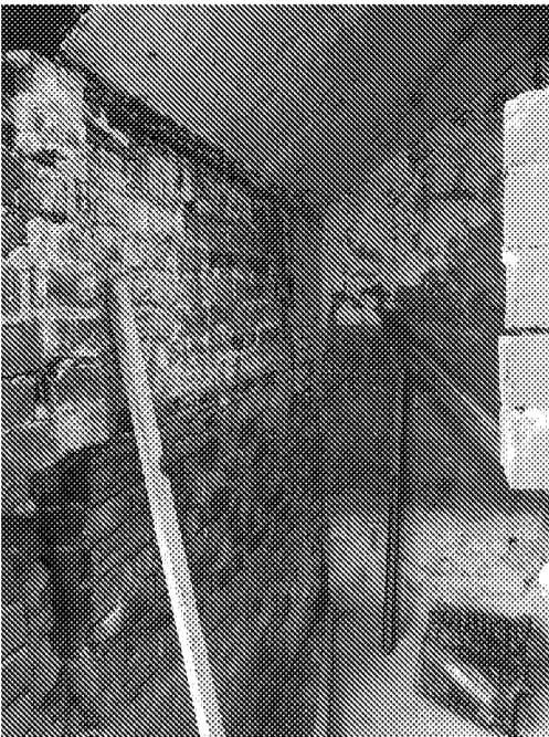
Photograph 2.02 The original floor has been replaced with a cementitious screed as part of a previous renovation and the inner wall finish is fair-faced brickwork and timber inserts.
