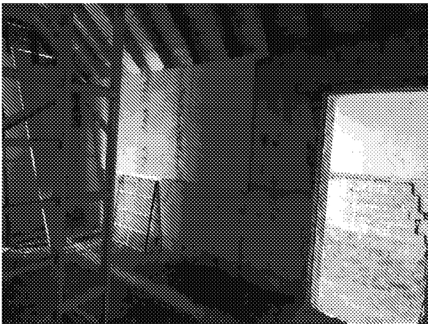
Photograph 1.02 Existing window opening boarded over, internal plastered finishes retained
