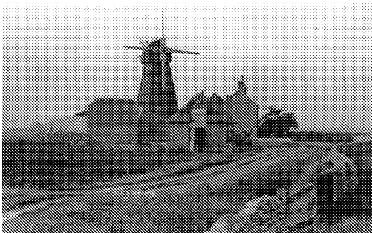
Plate 5a Thatch Barn south elevations with timber boarding and large shutters/doors c. 1910
