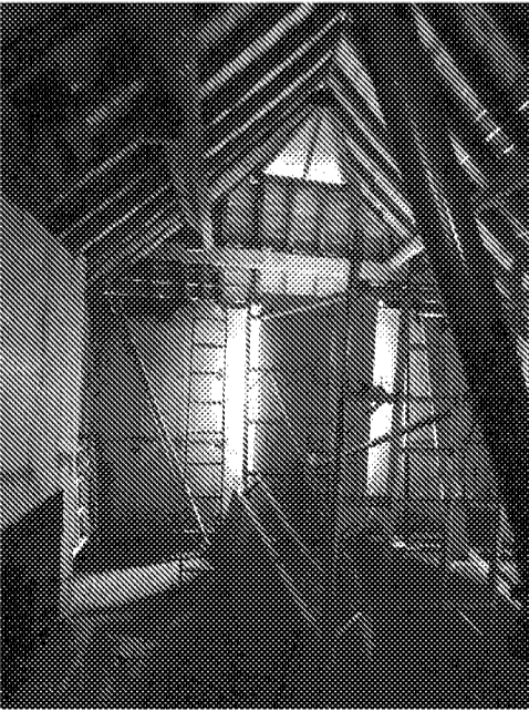
Photograph 1.02 Existing window opening boarded over, internal plastered finishes retained
