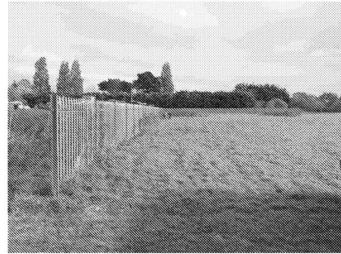
Existing fencing to southern boundary
