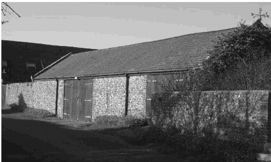
Figure 5 slate roof on flint garage
