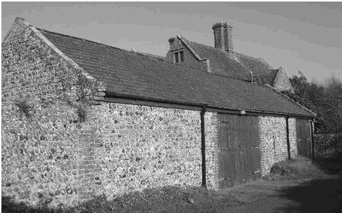
Figure 7 slate roof on flint garage Brookpit lane
