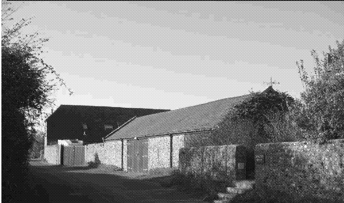
Figure 6 slate roof on flint garage Brookpit lane
