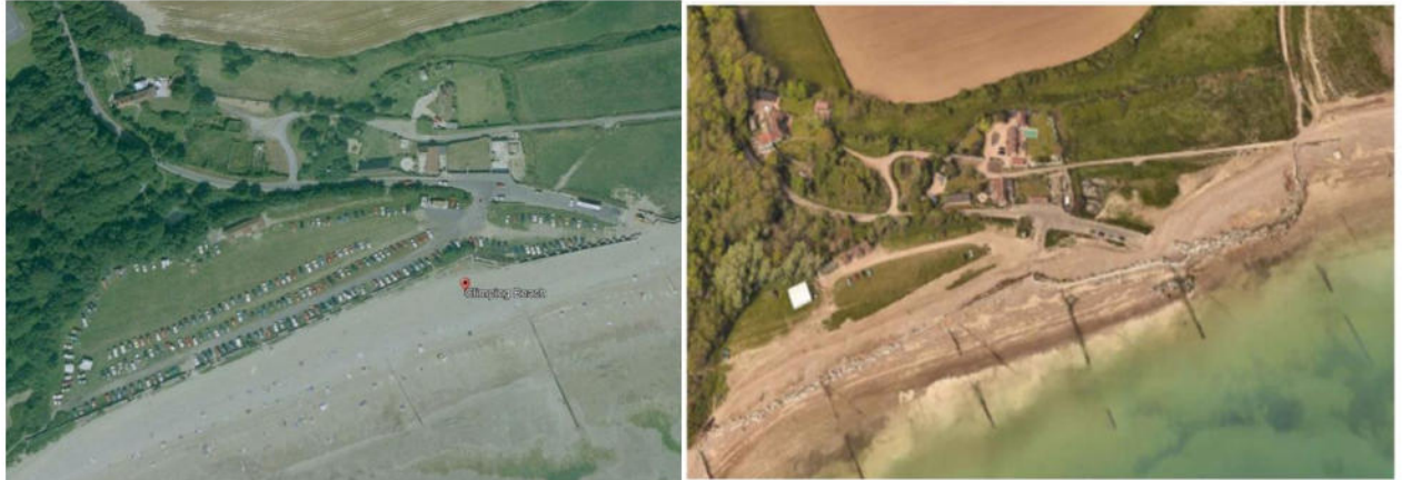
Figure 3. Aerial views of existing site indicating position and extent of erosion of car parking facility
