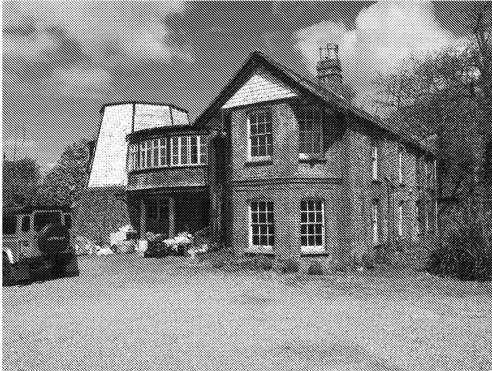
Figure 3 – Front of Mill building
