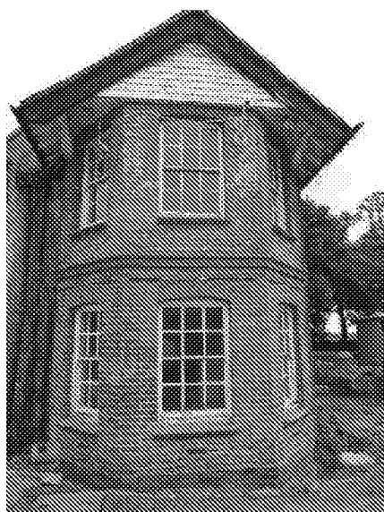
DSC03143 Double Height Canted Bay
