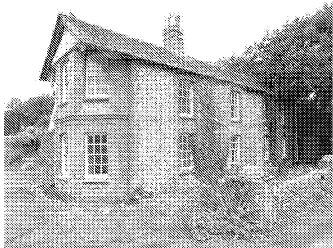
DSC02718 East & South Elevations, view looking North West
