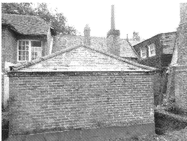
DSC02699 West Elevation
