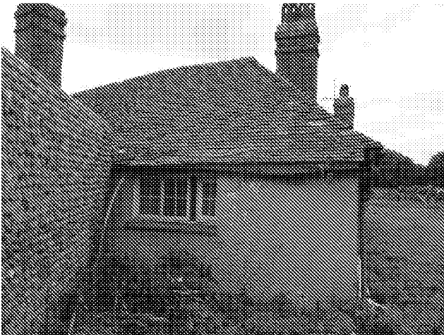
DSC03219: Western linear extension to Historic core of Mill Cottage, North Elevation
