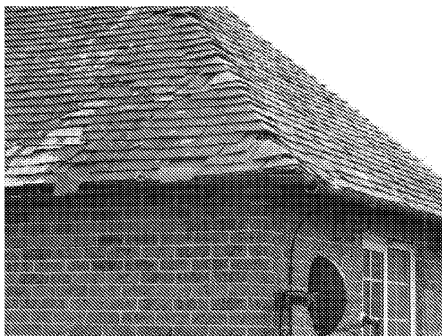
DSC03207: View of West Elevation Mill Cottage
