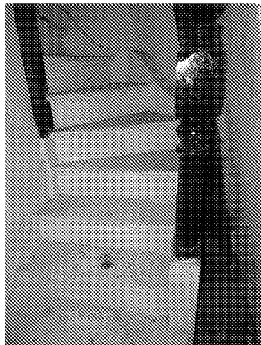
DSC02923 Existing staircase
