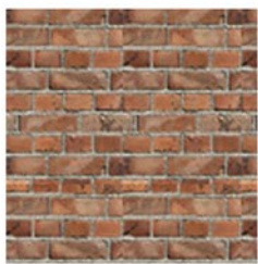
20th Century Brickwork
