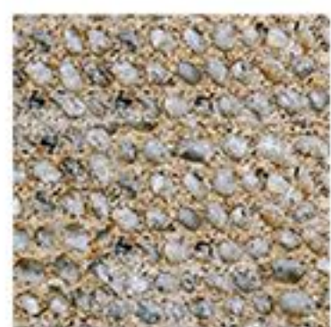
Traditional Flint Stone Wall
