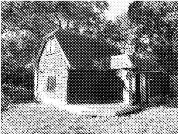
The building viewed from the south east
