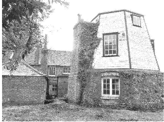
DSC02733 General view
