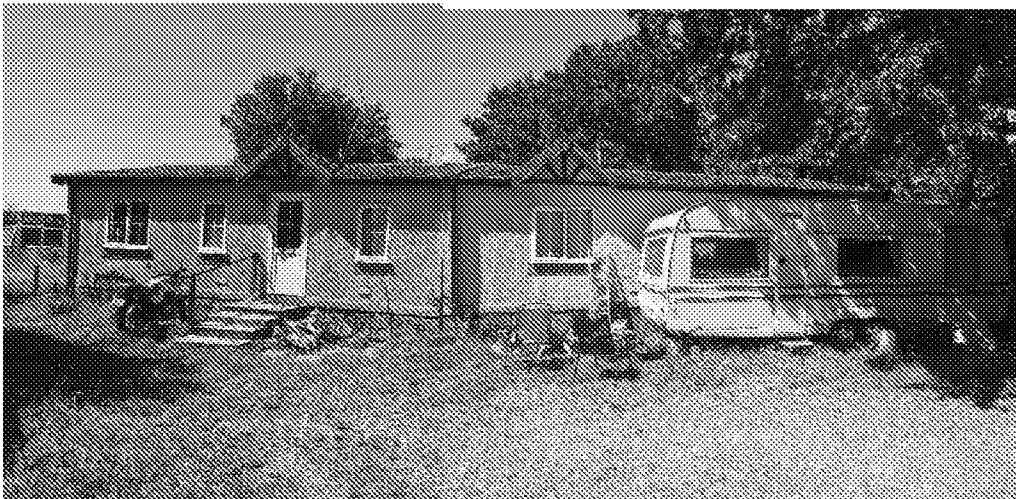
DSC03273 & DSC03274: Pre-fab building immediately to the west of Climping Mill to be removed. Elevation facing the mill.
