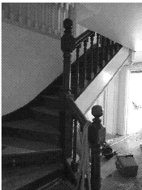
DSC02848 Main Stair
