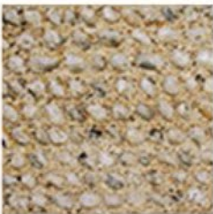
Traditional Flint Stone Wall
