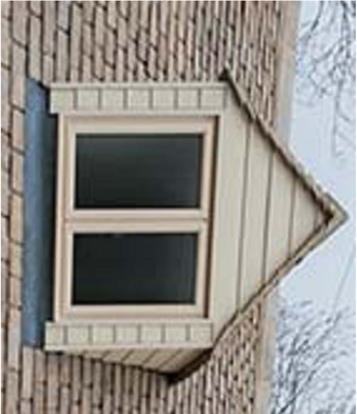
Fenestration: Cream Aluminium Windows externally, white inside
