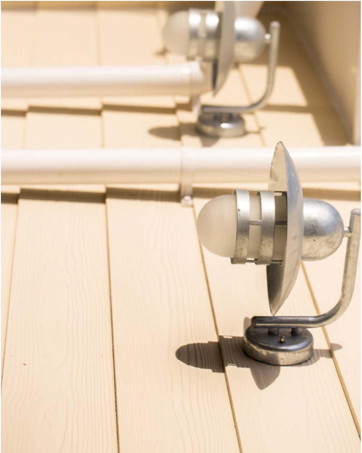
Weatherboarding: C02 Beige Cedral Fibre Cement lap boarding
