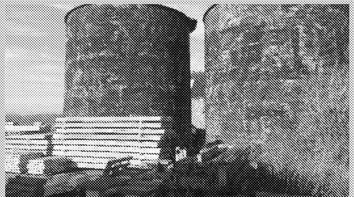
Photo 4: Disused grain silos.
