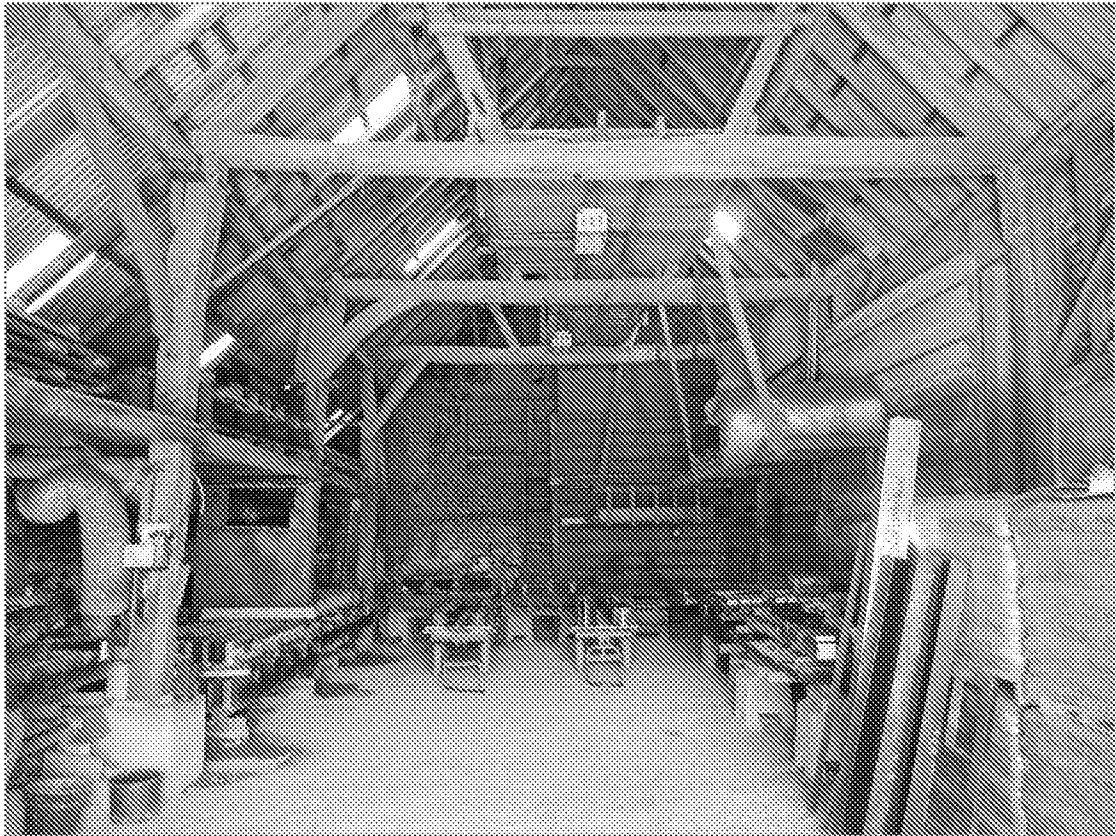
Figure 15: Barn interior, looking north
