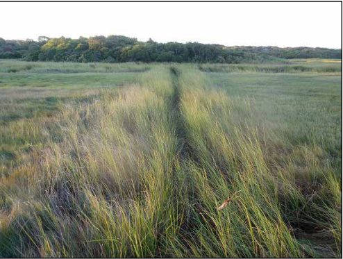
Ditch with vegetative growth
