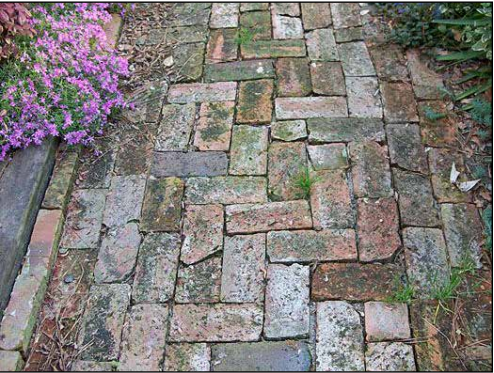
Patio Surface Recycled Bricks with sand filled joins
