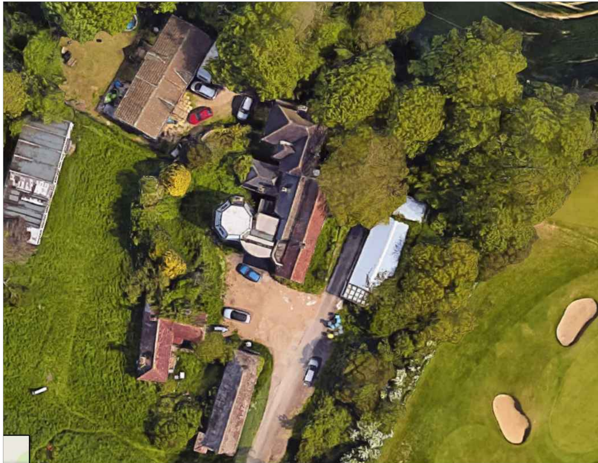
Aerial Image showing the varying roof coverings of Mill House, Kitchen Range, 1950's extension and The Mill
