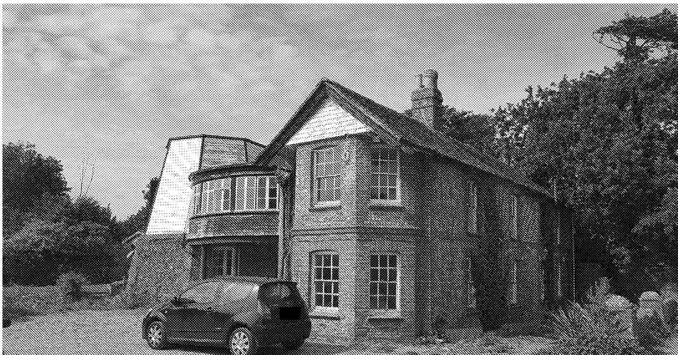
Photograph No. 1 - View of Building B1, assessed as providing High bat roost suitability.
