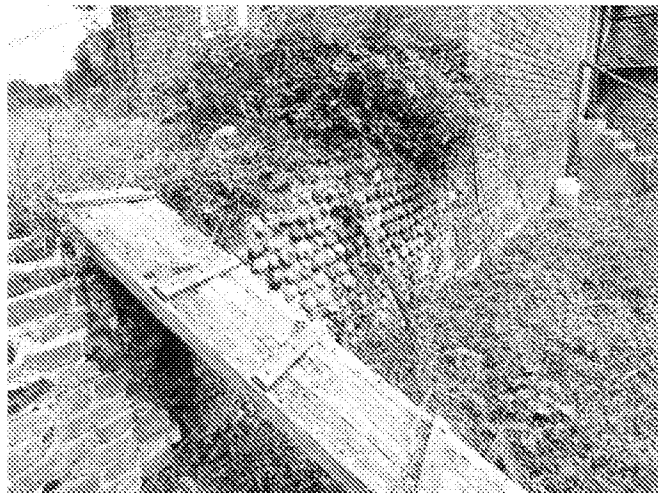
DSC02760 & DSC02762: Partial collapse and rebuilt section of garden wall to the South of Mill Cottage
