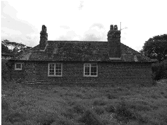
DSC03206: View of West Elevation Mill Cottage
