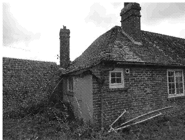
DSC03199: Former doorway infilled, West Elevation
