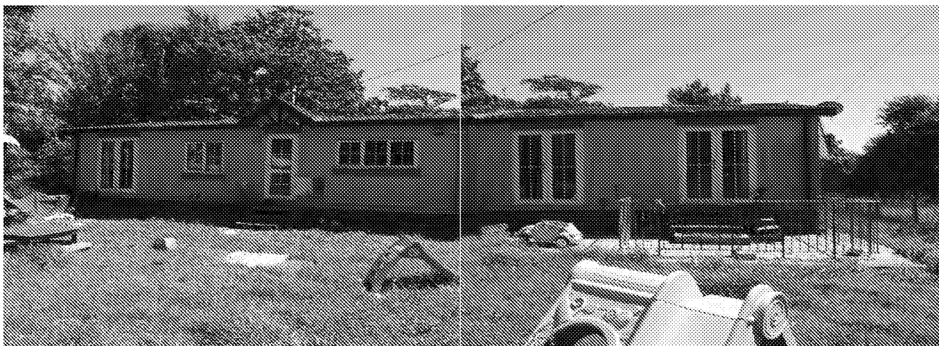
DSC03273 & DSC03274: Pre-fab building immediately to the west of Clymping Mill to be removed. Rear elevation
