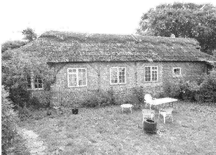
DSC02770: View of West Elevation, Mill Thatch
