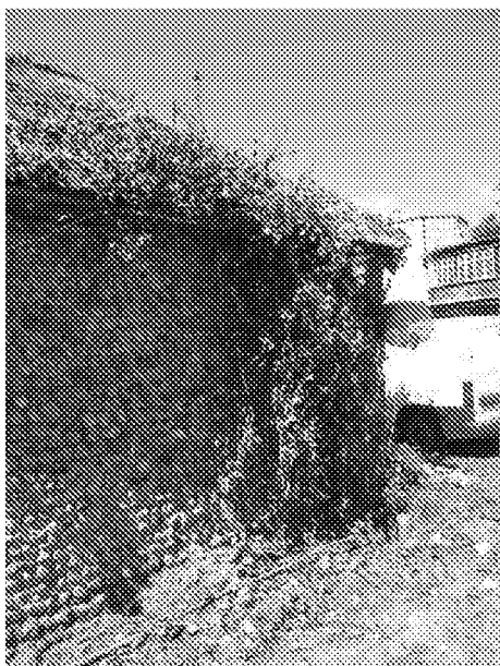
DSC03250: Established vegetation to East Elevation Mill Thatch No1
