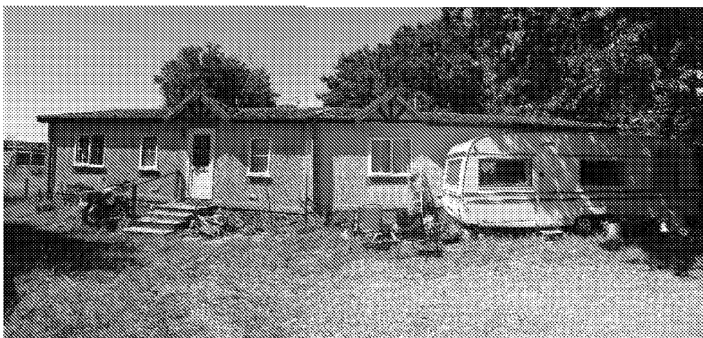
DSC03273 & DSC03274: Pre-fab building immediately to the west of Clymping Mill to be removed. Elevation facing the mill.
