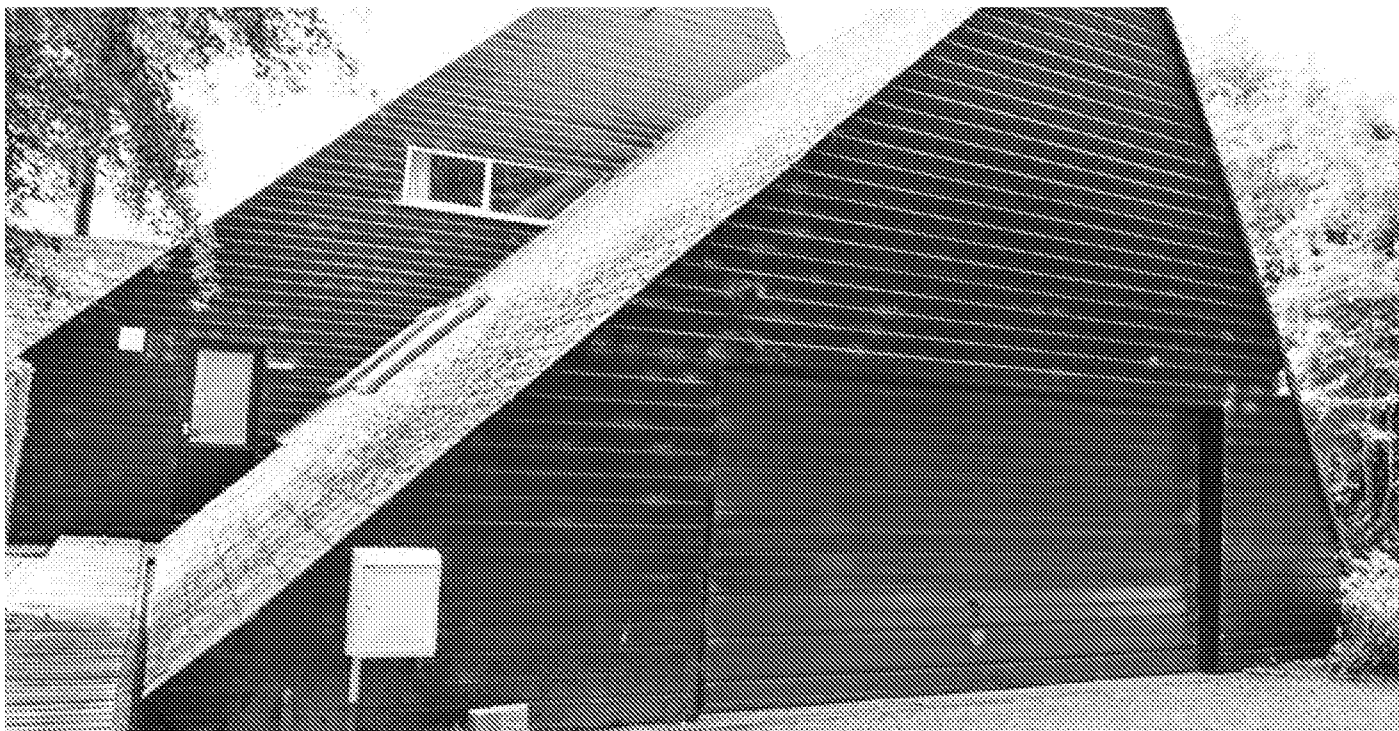
Photograph No. 05 - The garage structure consists of 2 no. windows on the eastern side, tightly sealed into the roof and tiles with little or no gaps around them.
