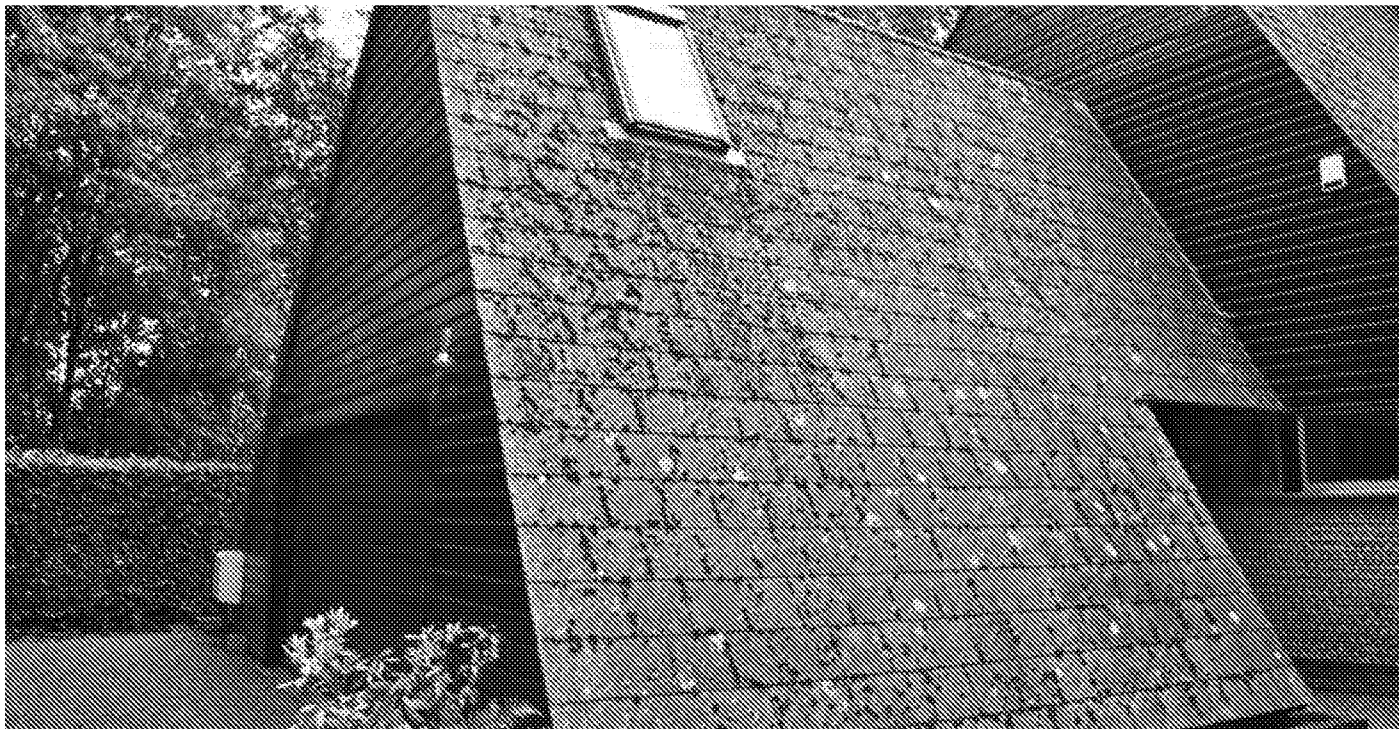
Photograph No. 03 - The tiles are made of thin concrete material with very little or no gaps between one another. The smaller ( garage ) structure contains; 1 no. window on the western side, tightly sealed into the roof and tiles with little or no gaps around it. The northern aspect consists of wooden sidings and metal garage door.
