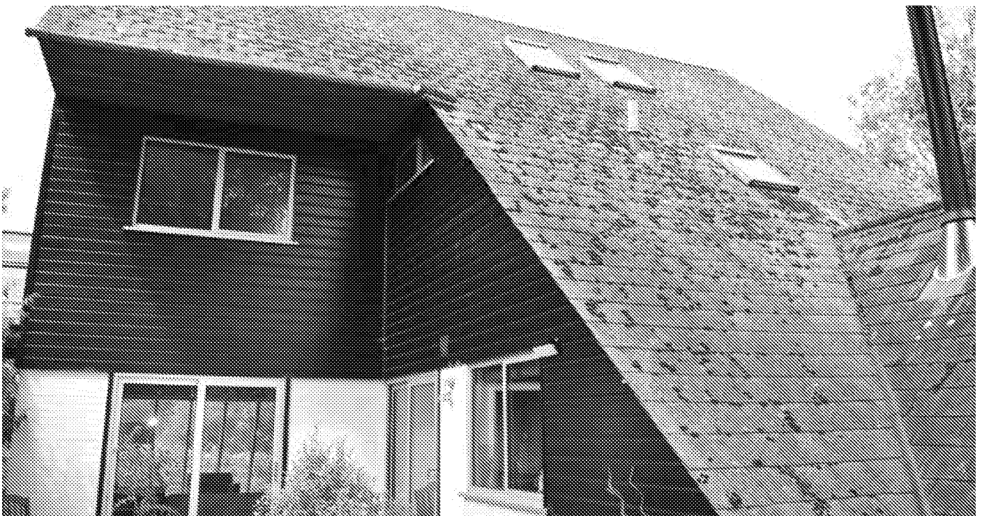
Photograph No. 08 - The eastern aspect of the property covers many angles and edges, all have limited potential for bat roosts.
