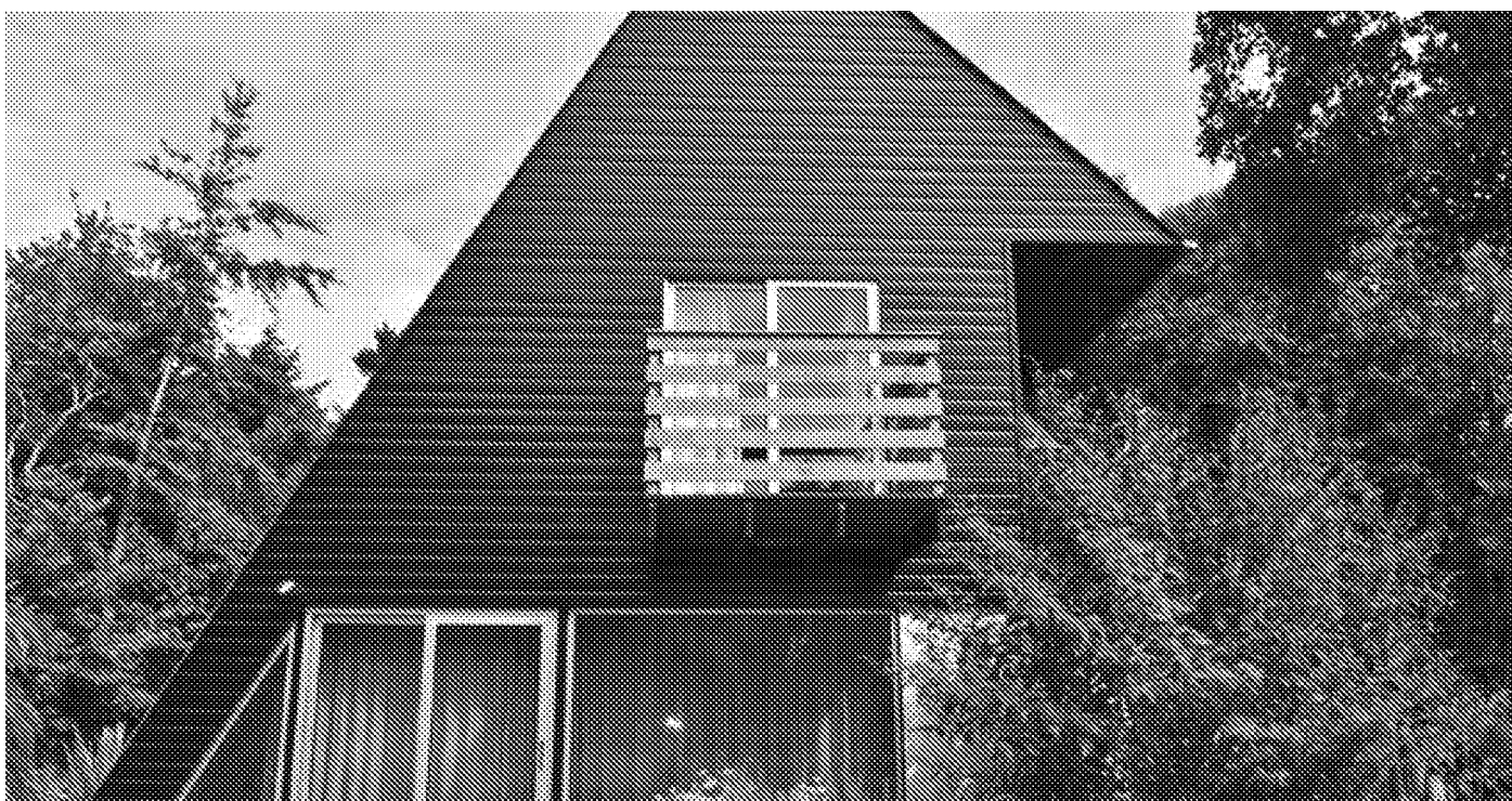
Photograph No. 10 - The southern aspect is covered in wooden sidings with small balcony and patio doors fitted tightly against the wooden frames. No visible gaps suitable for bat roosts were noted.
