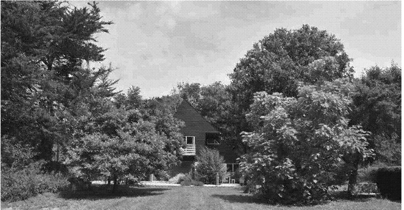
Photograph No. 01 - Southern aspect of the existing residential property with adjacent amenity lawn and scattered trees, the building is of a bespoke architectural design.
