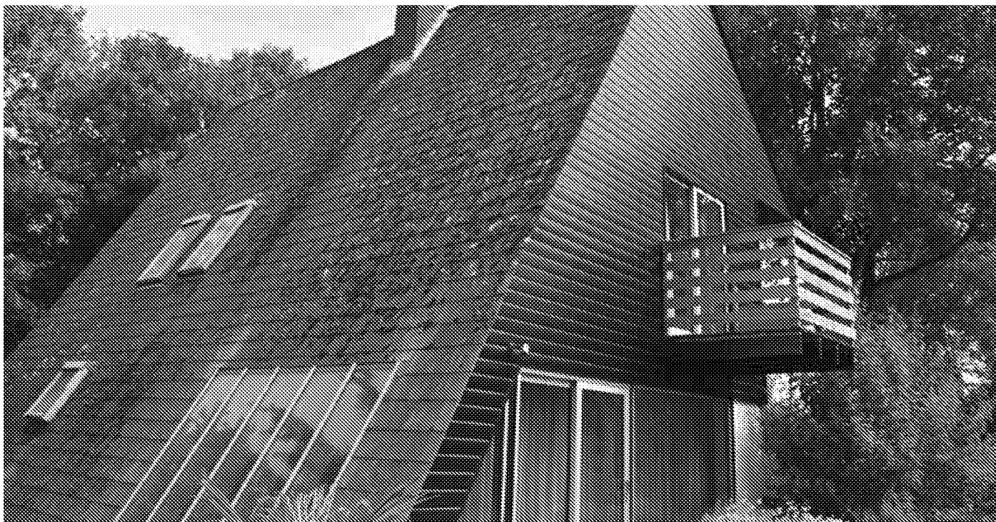
Photograph No. 09 - The main house structure on the western aspect is covered in mainly concrete tiles, with 4 no. windows. All of the windows are fitted tightly into the roof with no visible gaps suitable for bat roosting.
