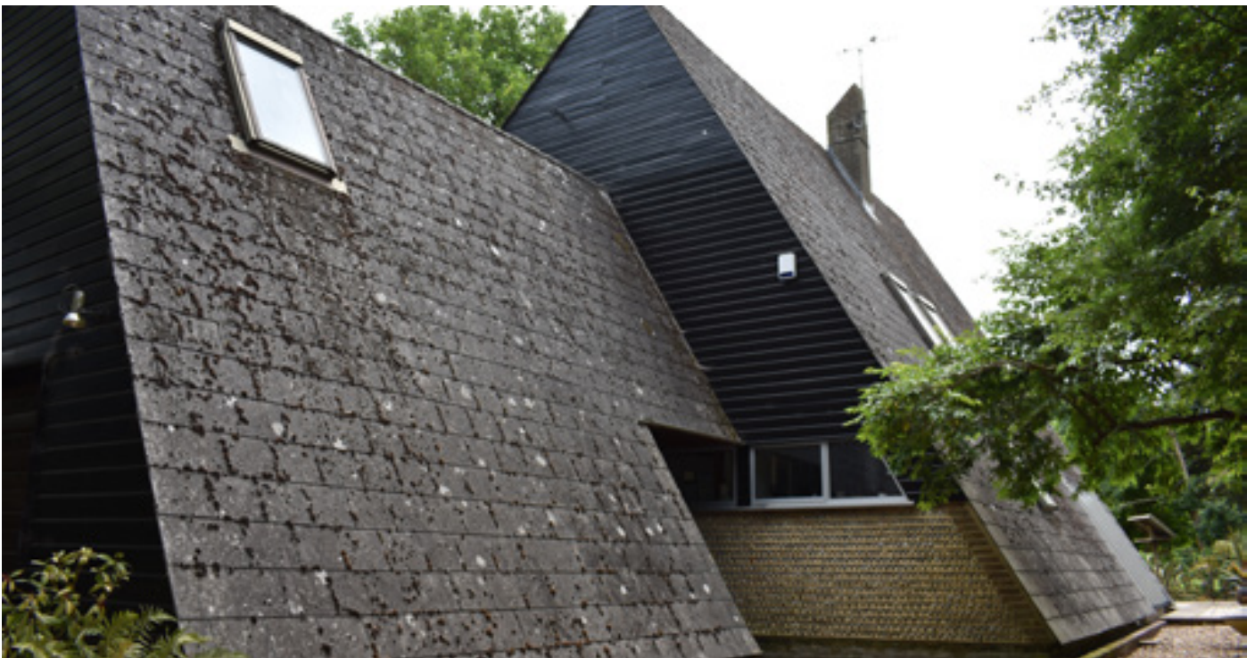
Photograph No. 02 - Formed of 2 no. triangular structures linked via the garage and main building. On the Eastern aspect ( shown ), the roof runs the entire length of the building, and sits within 10 cm of the ground.
