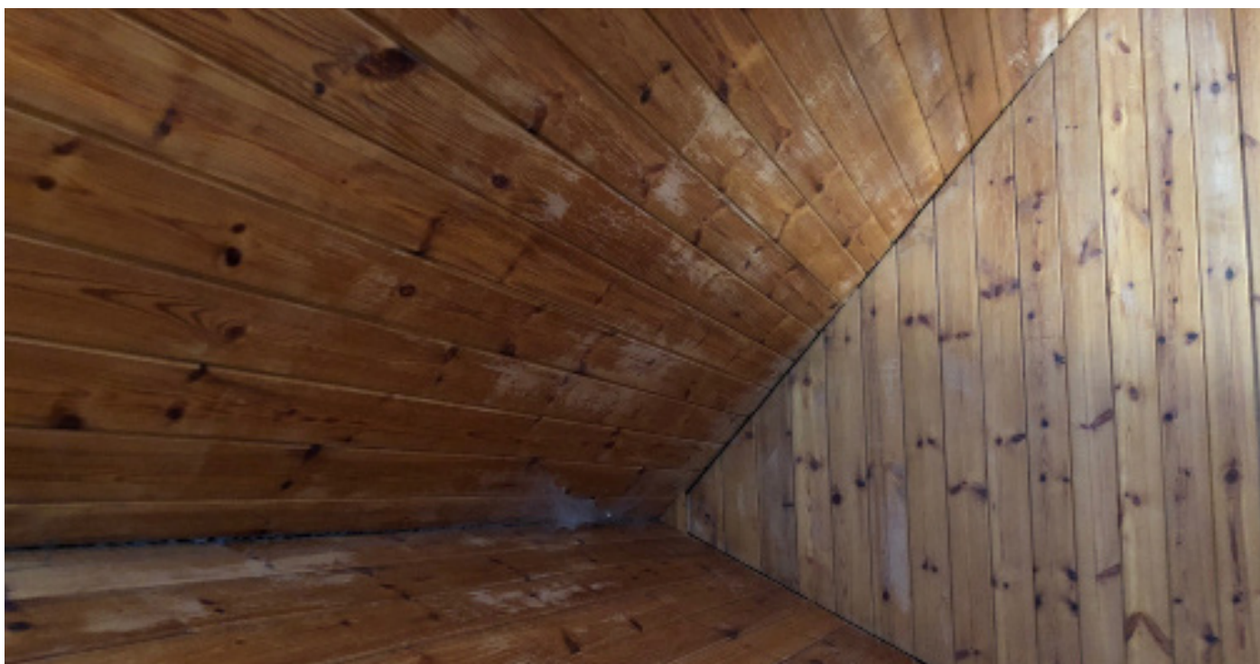
Photograph No. 10 - Inside the property there is no loft void. the ceiling height continues into the otherwise roof space.
