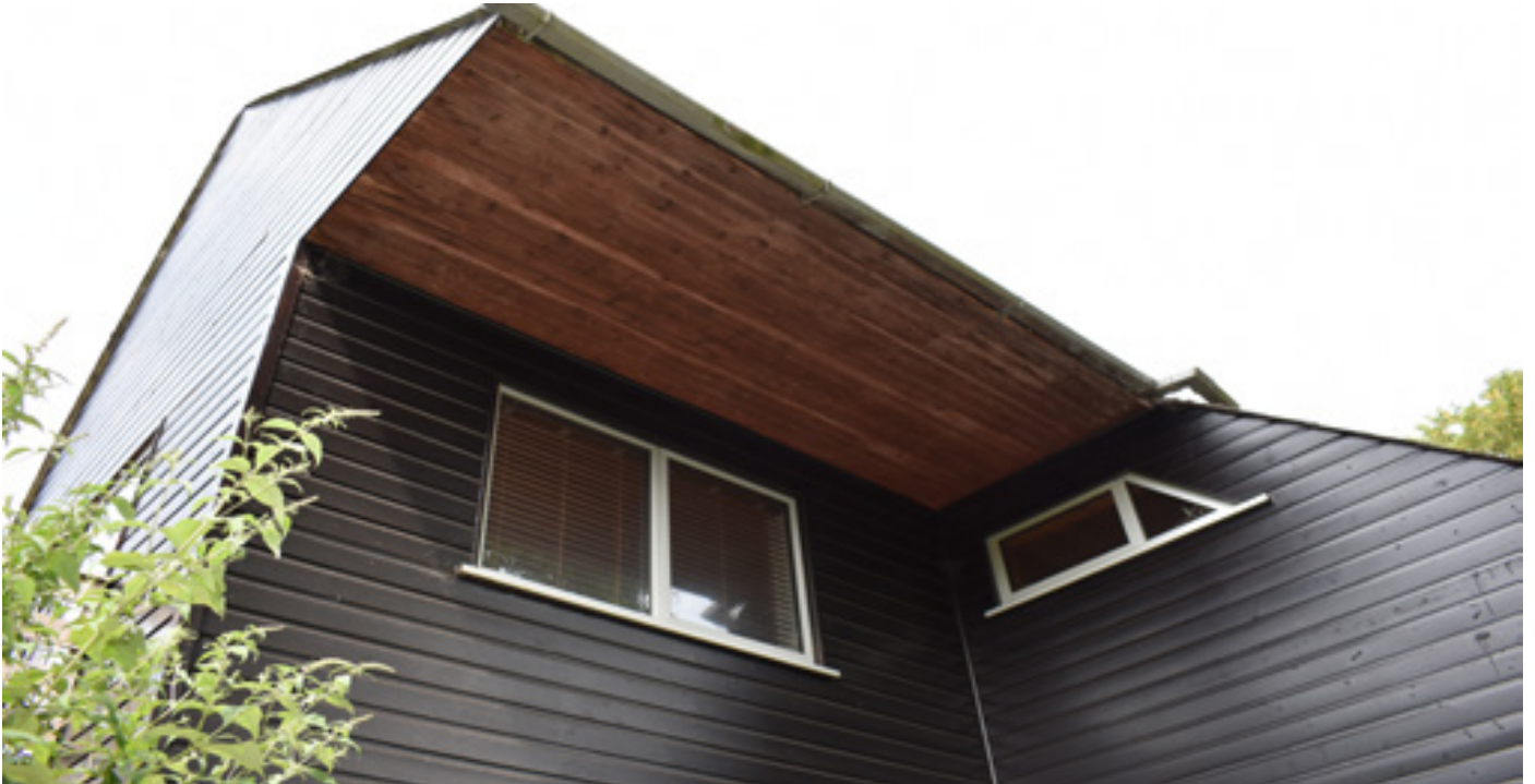
Photograph No. 07 - The wooden sidings on the eastern aspect were also noted as tightly fitted with no visible gaps suitable for bat roosting.
