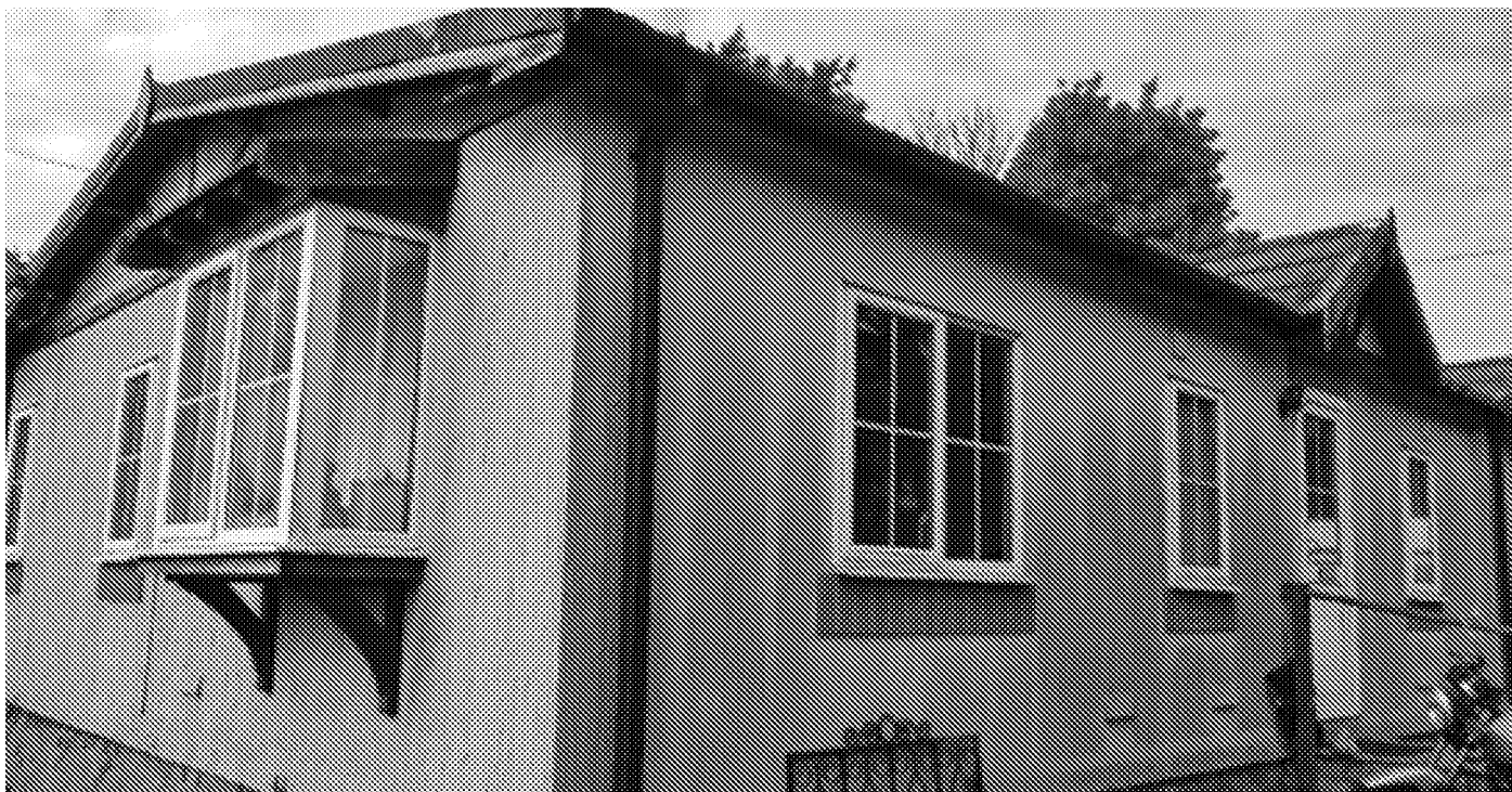
Photograph No. 5 - Building B5, assessed as providing 'negligible' bat roost potential.
