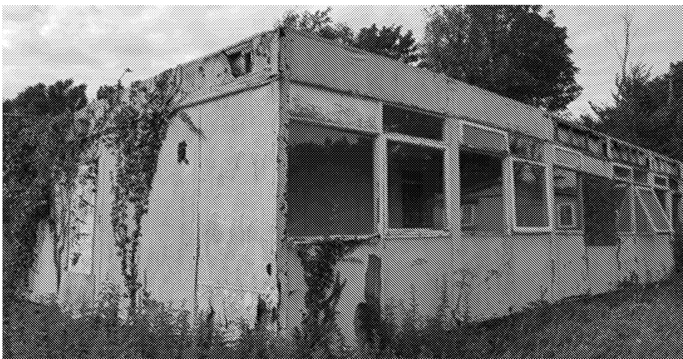
Photograph No. 4 - Building B4, assessed as providing 'negligible' bat roost potential.
