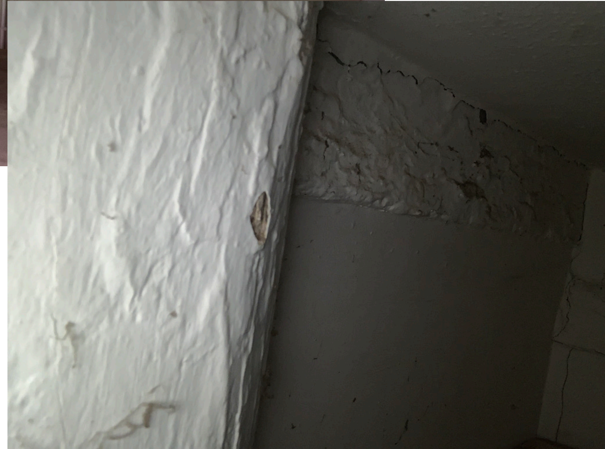
Original rear wall currently hidden in cupboards
