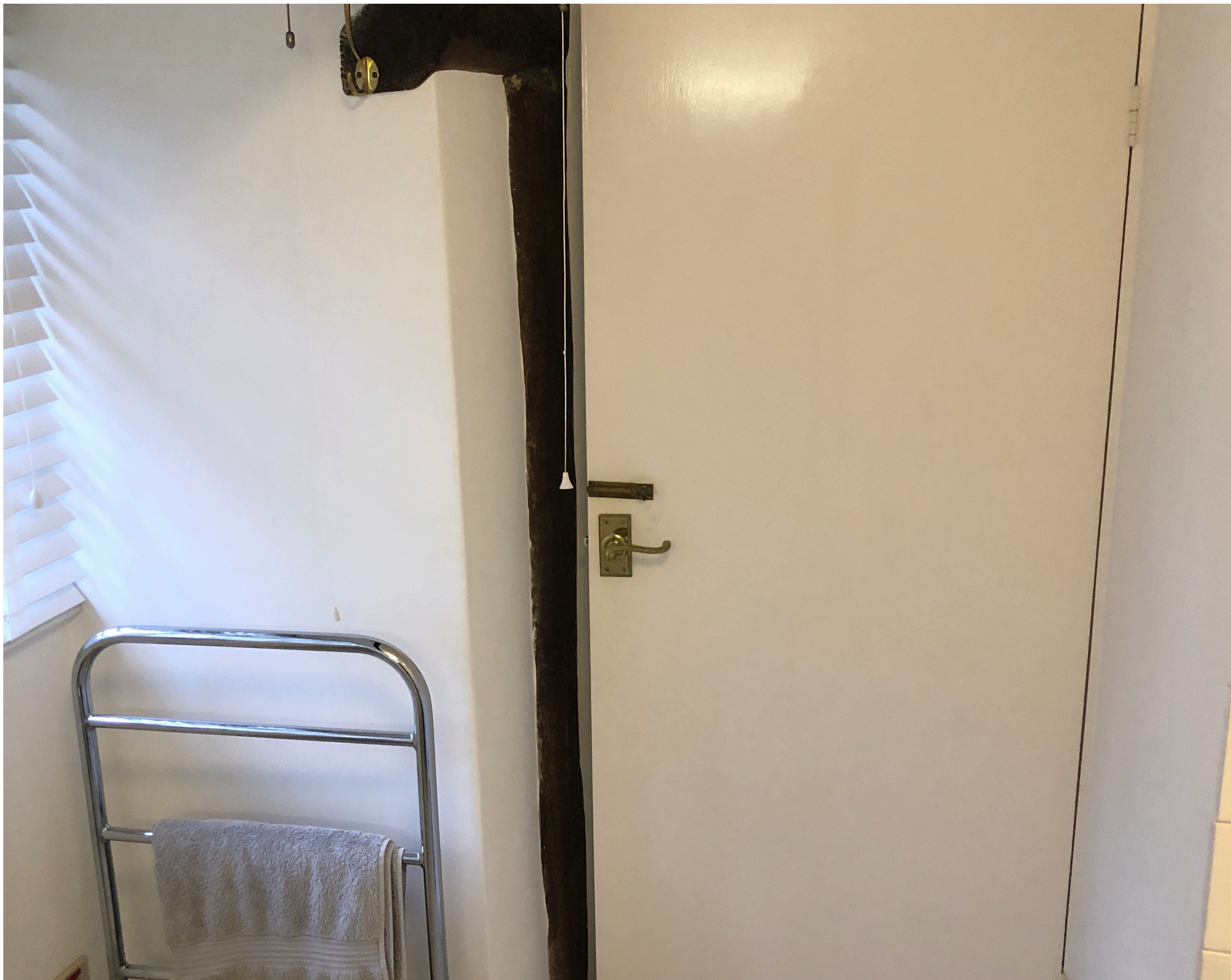
Existing hollow panel doors upstairs
