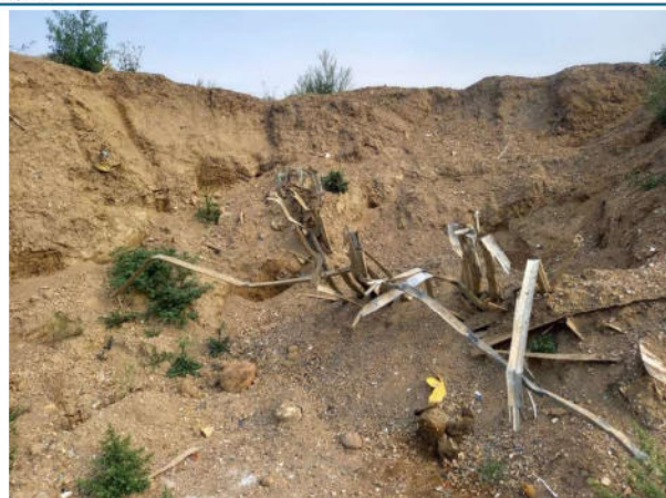
2. Materials in stockpile which encroaches onto site from the south
