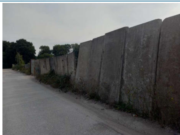
8. Site eastern boundary partly formed from reaction wall sections
