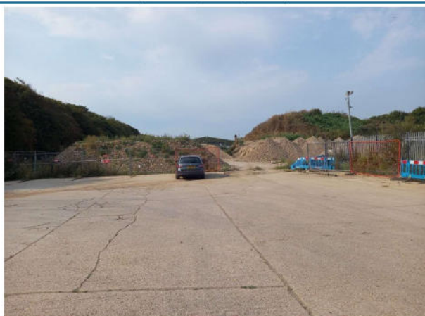
3. Northern part of the site comprising concrete hardstanding
