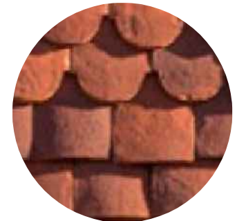
Upper Walls - Tile hanging
