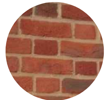
Lower Walls - Brick
