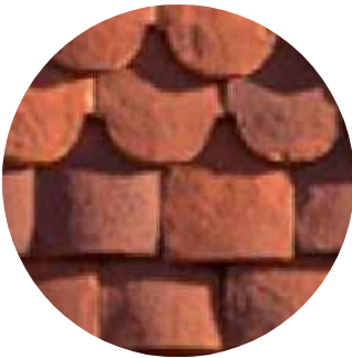
Upper Walls - Tile hanging
