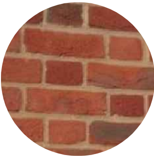
Lower Walls - Brick
