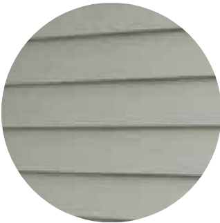
Upper Walls - Painted weatherboard
