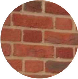
Lower Walls - Brick
