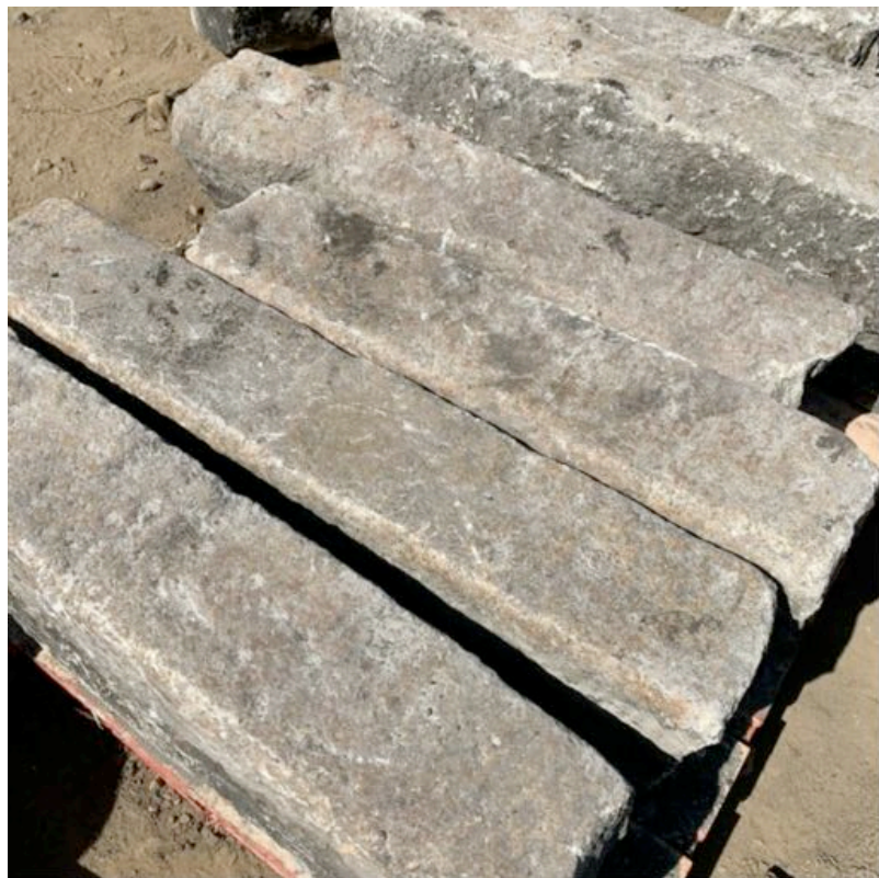
Locally sourced reclaimed granite kerb/ step stones, laid in hydraulic lime mortar.
