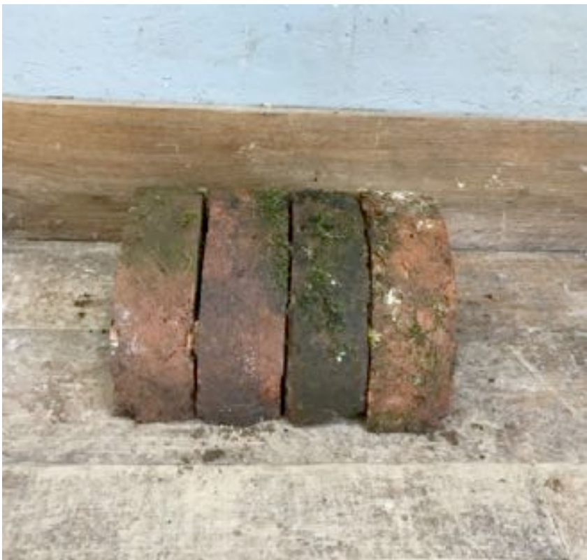
Locally sourced reclaimed "Half Round" bricks, laid in hydraulic lime mortar.
