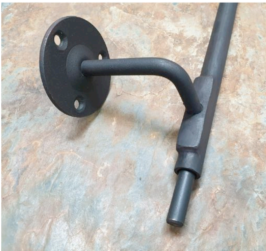
Handcrafted discreet wrought iron handrail fixed to inside of stone staircase. Not visible on elevation.
