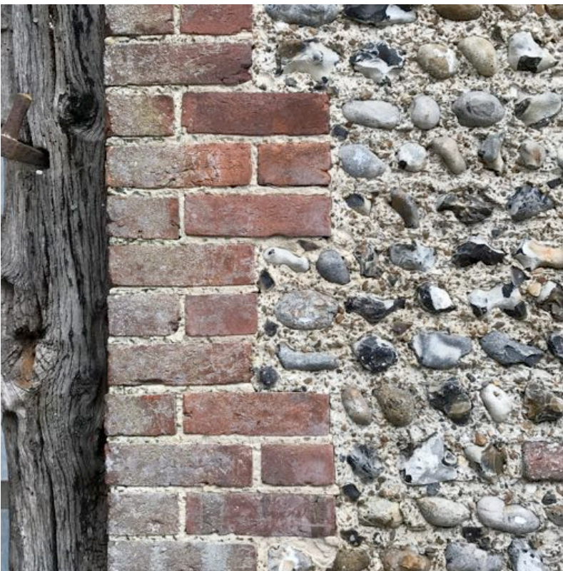
New brick quoining to match existing using locally sourced reclaimed bricks, laid in hydraulic lime mortar.
