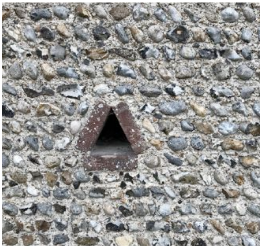
New flint work to match existing, laid coursed using locally sourced cobbled & napped flints, laid in hydraulic lime mortar.
