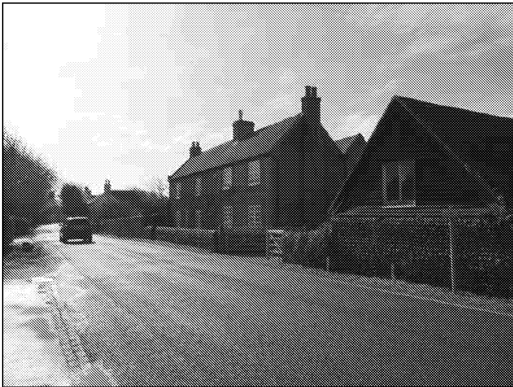
Plate 4 Dove Cottage (Grade II Listed, NHLE: 1233449)
