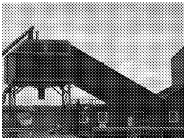
Figure 1 - Fully enclosed Conveyor
