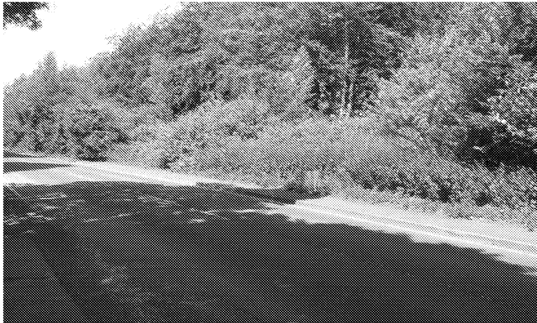
View looking north east across the Yapton Road towards the land
