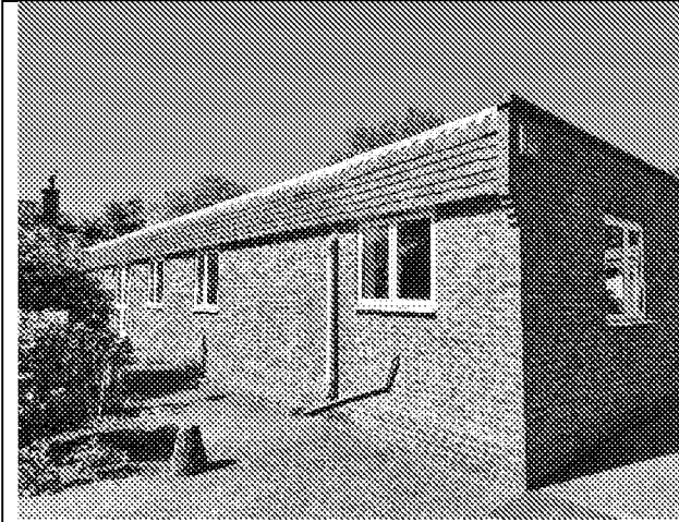
Photograph 1 – the residential flat viewed from the southern corner.
