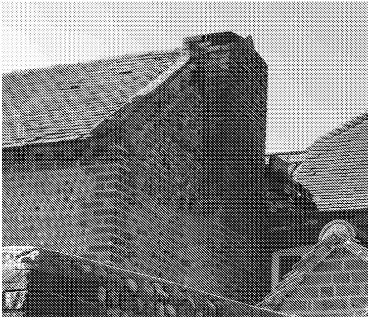
IMAGE OF EXISTING CONDITION
