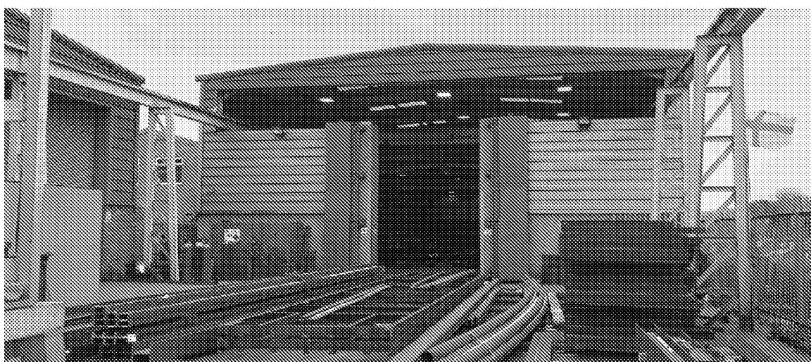
Figure 4: External Courtyard and Crane System
