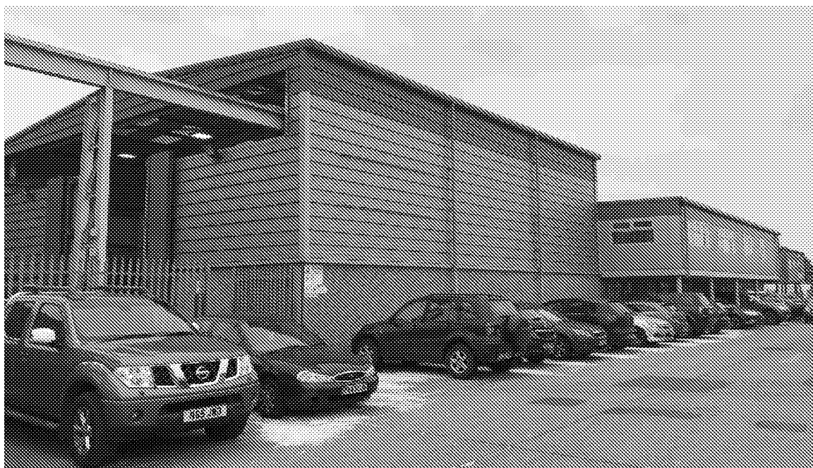
Figure 3: Workshop and Offices
