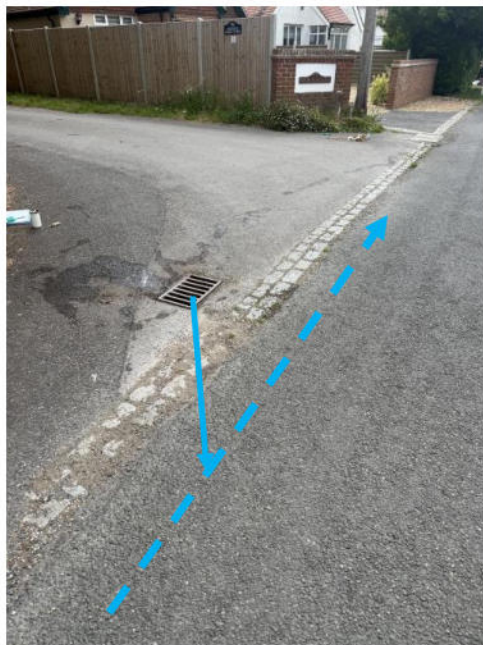
CCTV Survey was carried out on the road gully.
